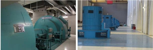
Fourteen pumps lift the water almost 2,000 feet over the mountains, where it is split into two aqueducts that serve Southern California.
